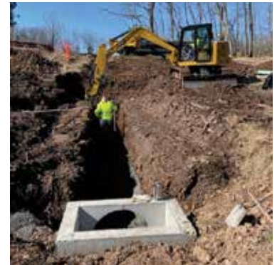
Enos Godshall Park – storm pipe & inlet being installed
