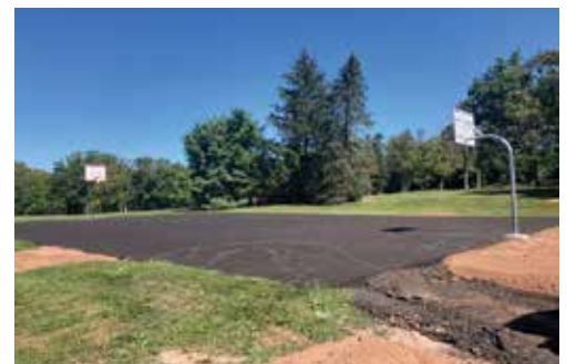
Branchwood Park basketball court under construction
