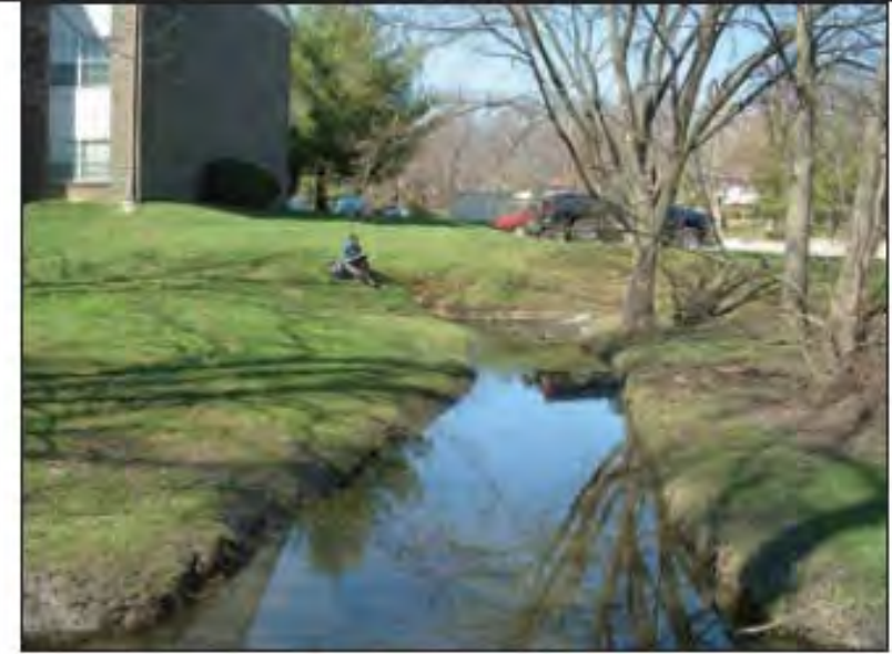
Fully submerged: Can't see outfall
