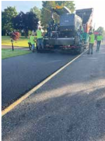
Ultra-thin overlay process being applied to Mininger Road
