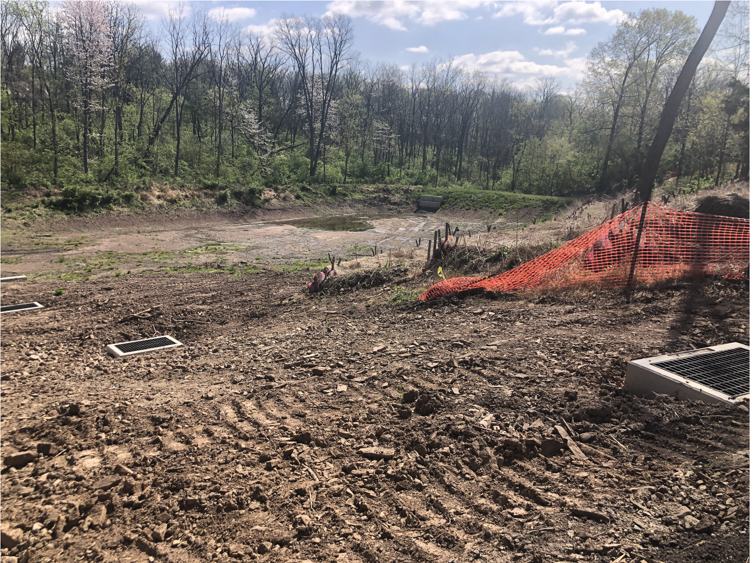
Enos Godshall Pond - Under Construction 2023
