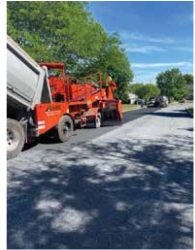
Double Seal Coat followed by Polymer Modified Fog Seal process
