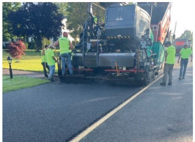
Ultra-thin overlay process being applied to Mininger Road. Double Seal Coat followed by Polymer Modified Fog Seal process
