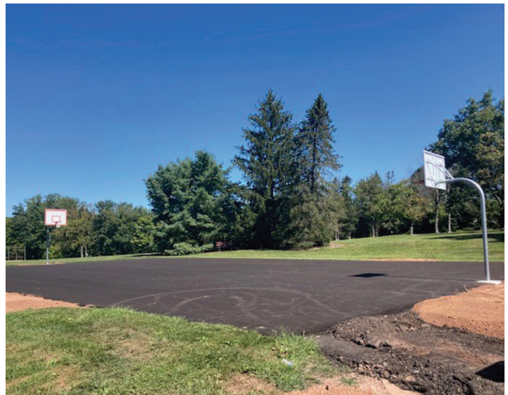
Branchwood Park basketball court under construction
