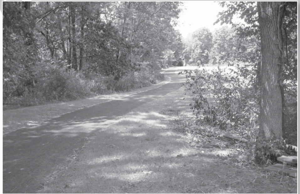
Newly constructed West Broad Trail.
